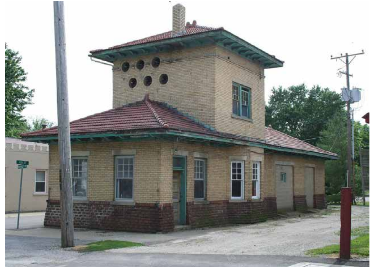
Old Bondville, Illinois interurban rail station and power plant, 2007.
