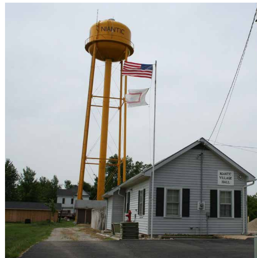
Niantic Village Hall and water tower.
